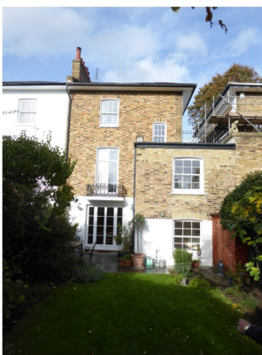
Rear elevation (North) and garden
